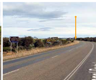
Advance warning for Stokes National Park are in need of improvement, especially for west bound motorists as the turn-off to Stokes NP is at the end of an overtaking lane and on bend in the highway.
