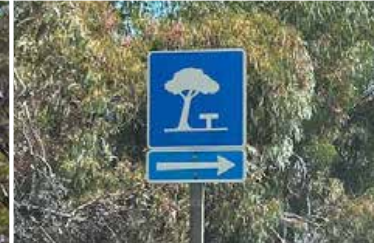
Salmon Gums - well appointed rest area with advance warning and a mix of directional signs. Directional signs should be consolidated, trees cut back and the signs positioned on the correct side of the road.
