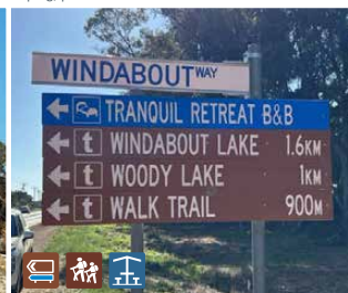
Fisheries Rd/Windabout Way intersection - Too much information, this intersection should have a double sided brown directional sign "Woody Lake Reserve" and the appropriate AS symbols. B&B sign should be below.
