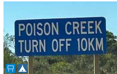
This sign should be replaced with a blue advance warning sign and the AS symbol for camping.
