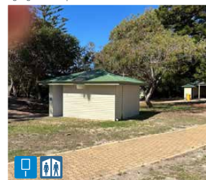
Dempster St - Install double sided public toilets positional signage adjacent toilets.
