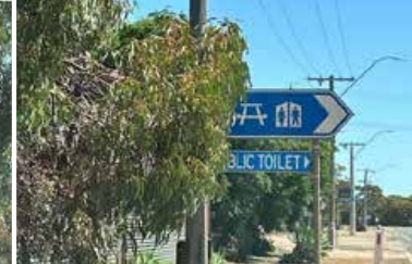
Salmon Gums - well appointed rest area with advance warning and a mix of directional signs. Directional signs should be consolidated, trees cut back and the signs positioned on the correct side of the road.
