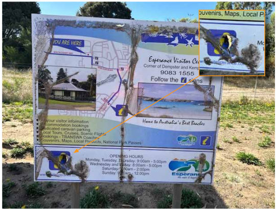
South Coast Hwy - Poorly produced ancillary sign promoting the Esperance Visitor Centre, vinyl has failed and there is a large hole in the bottom left-hand corner
